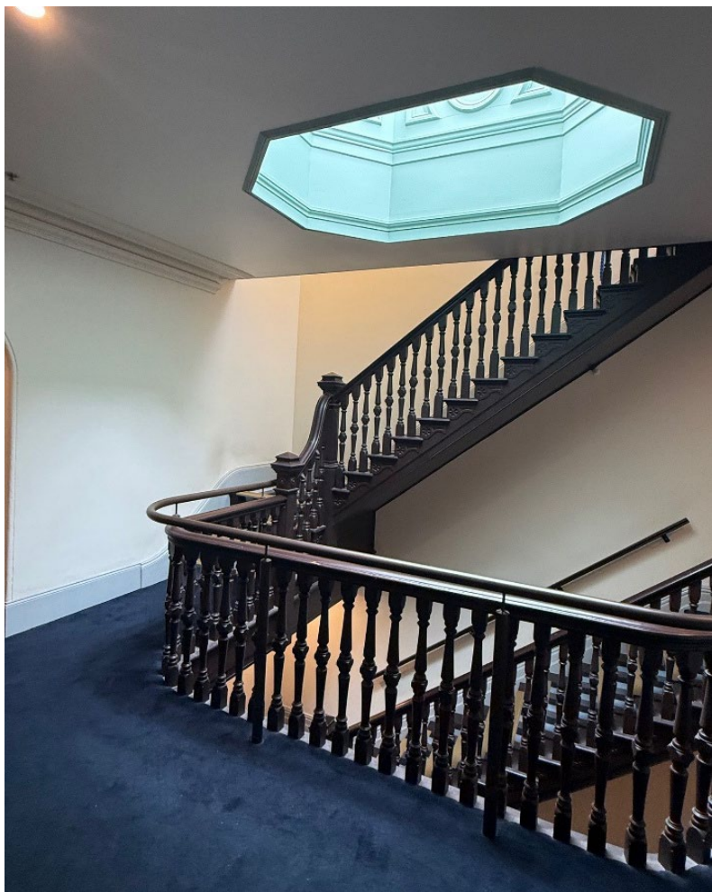
existing stair access to the rooftop
